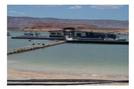
This small diesel tank sits between the 2 larger gasoline tanks. Each tank has its own independent enclosure within the floating tertiary containment structure. The ASTs are filled from a shoreside tanker through a loading manifold on the beach which is equipped with spill containment and doublewalled piping to the ASTs.
